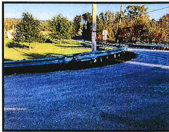
Figure 3: Damaged Guiderail on the Left Side of Cannery Road
