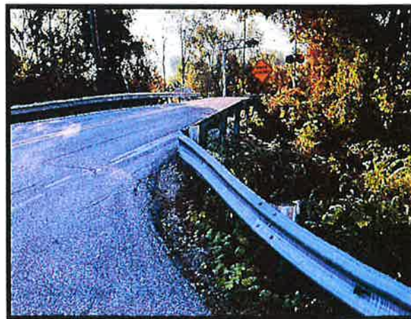
Figure 4: Damaged Guiderail on the Right Side of Cannery Road
